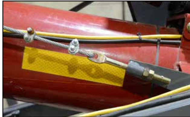
Fig 45 - Adjusting eyebolts at bottom of cable
